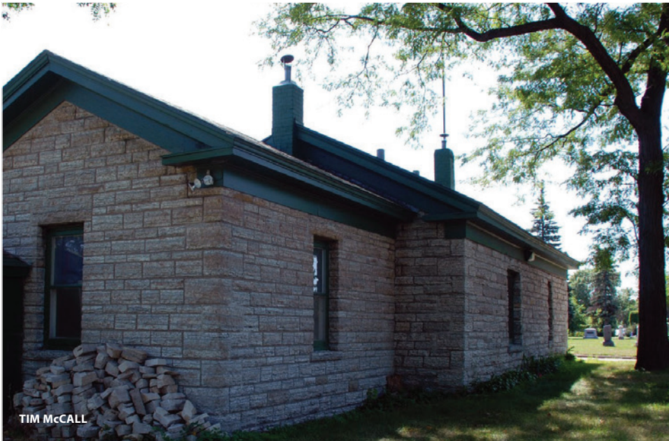
Caretaker Cottage 1940 masonry straight-cut edges differ with 1871 hand-chiseled. One of five Phillips buildings on the National Register of Historic Places.
