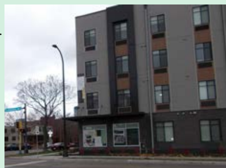
Park and Franklin Lofts
