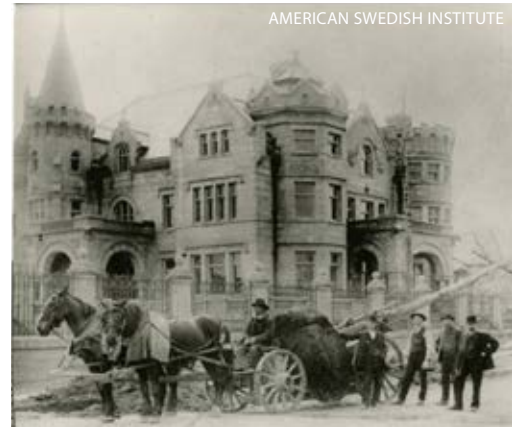
Tree delivery by horse-drawn cart next to Swan J. Turnblad residence, 26th Street, Minneapolis, Minnesota. Completed in 1908, the Swan J. Turnblad mansion was built in the French Chateausque style. The house became the American Swedish Institute in 1929.
