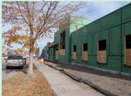
Community Care Clinics construction
