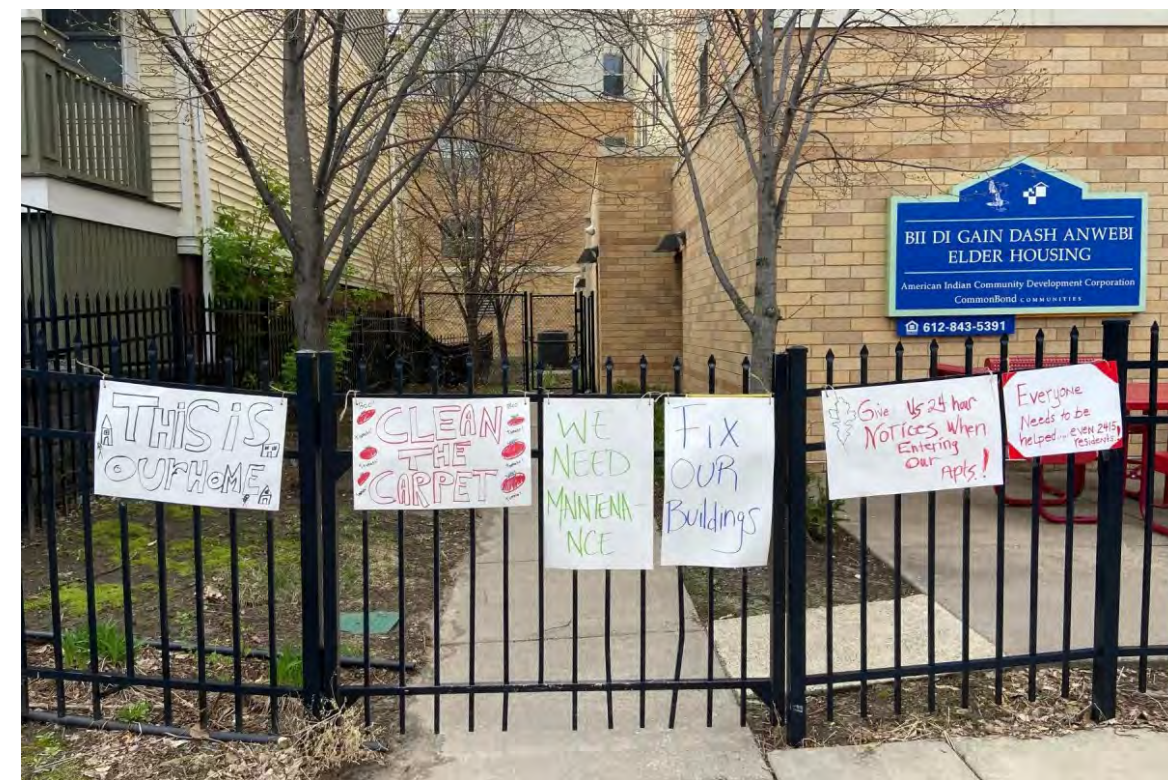
Signs posted on the gate of the Bii Di Gain Dash Anwebi affordable housing apartment complex in south Minneapolis on May 1, 2024, demand better living conditions.
