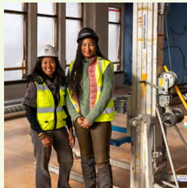
Project collaborators Alicia Belton of Urban Design Perspectives and Taylor Smrikárova of Redesign, Inc. at the renovation jobsite.
