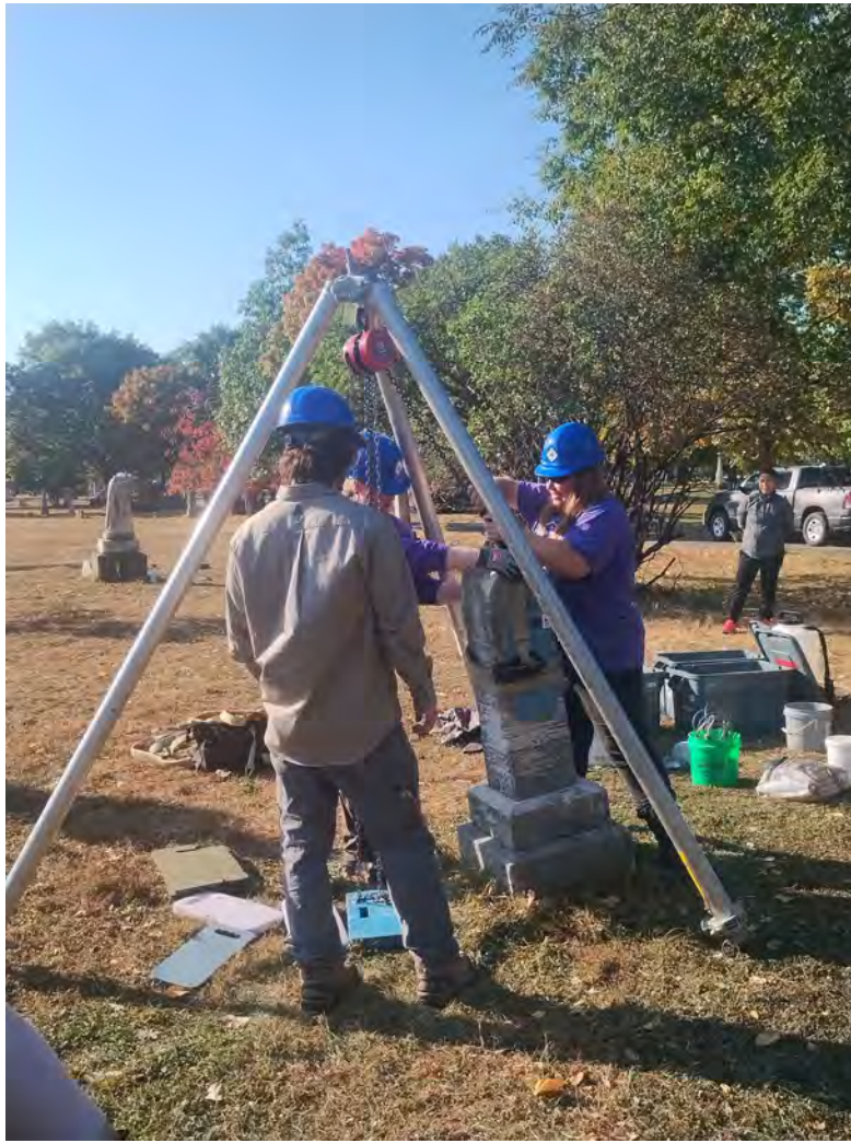
Northern Bedrock staff resetting and stabilizing the marker of Solomon Hare, African-American Civil War veteran and Buffalo Soldier.
